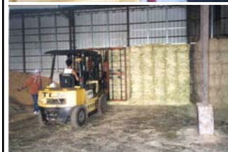
Inside of the covered, steel pole barn used to store bags of DDGS and other forage and feed ingredients at LFY Dairy.
